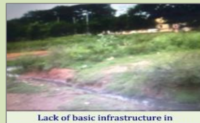
Lack of basic infrastructure in Chenchupeta Township, Tenali (April 2011)
