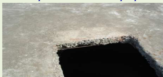
Sump without water vents
