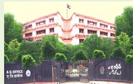
Offices of the Accountants General, Andhra Pradesh
