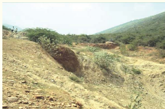
Eastern Main Canal at Km 6.00 to 10.00 delayed due to non acquisition of Forest Land
