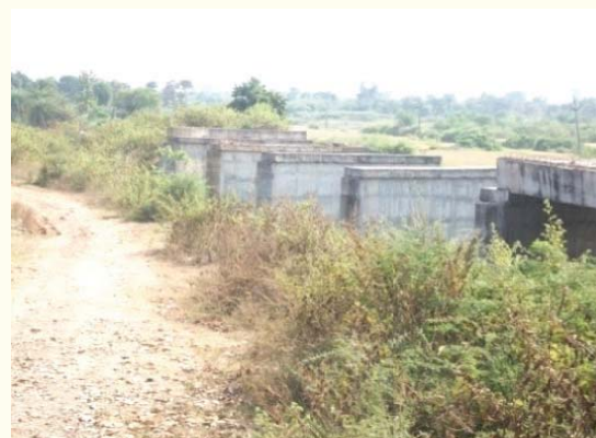
Incomplete bridge at Km 24.284 of FFC (Package-88)
