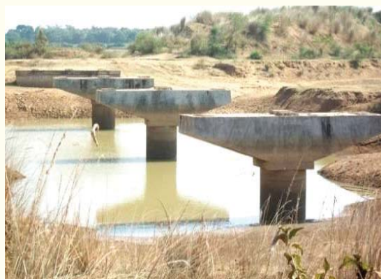
Incomplete bridge at Km 13.062 of FFC (Package-87)
