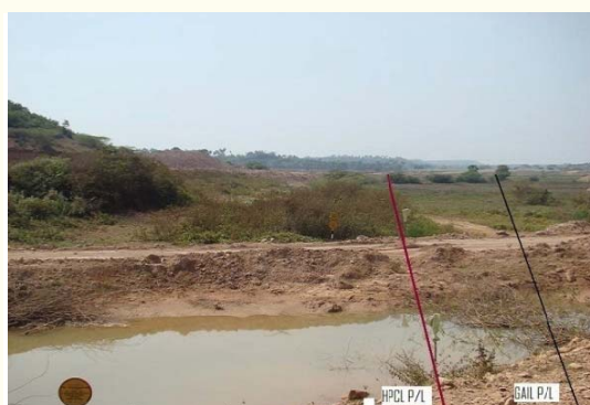
Untackled portion of ISRMC due to HPCL-GAIL crossing (Package 2)
